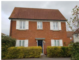
Existing detached house opposite
